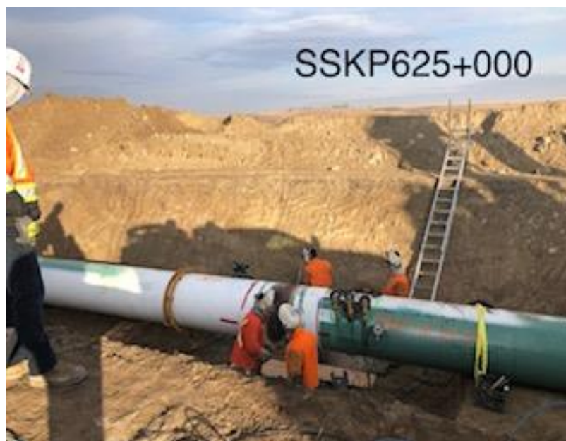
Welding a joint section main line
