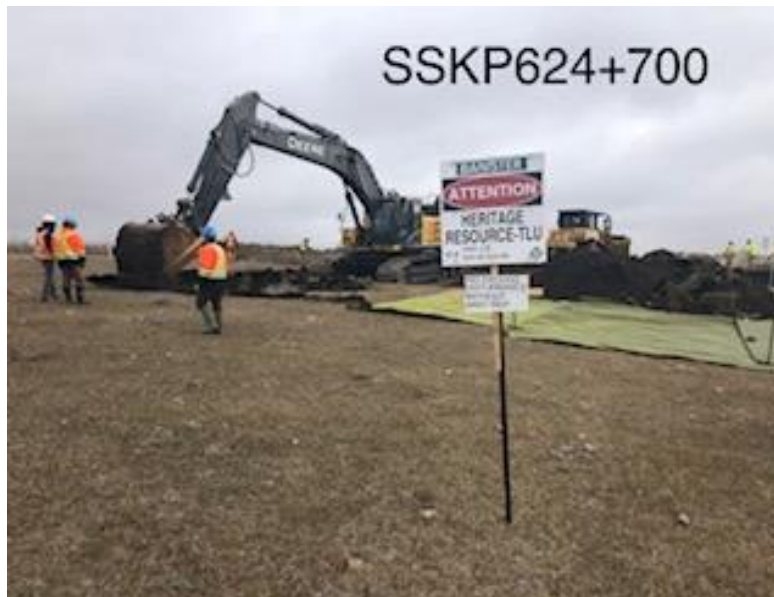
Topsoil excavation HDD entry point SSKP624+700
