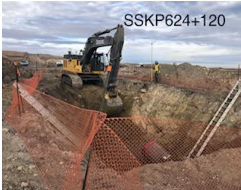
Bellhole excavation HDD exit SSKP624+100
